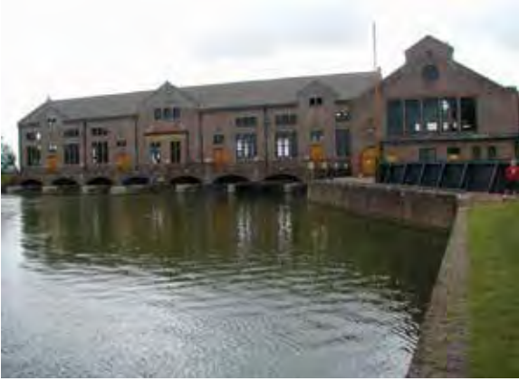
Figure 17.13. Left: the Wouda pumping station was built to drain large areas in Friesland, Netherlands, and is the largest steam pumping station ever built. It is now on the World Heritage List. Right: A drainage ditch removes excess water and lowers the water table in newly developed lands (“polders”) in the Netherlands.
