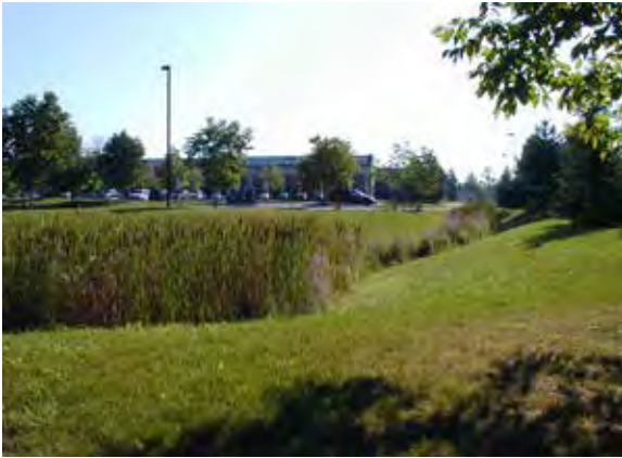
Figure 22.8. Retention of urban stormwater. Left: A swale that contains runoff from a parking lot in the distance. Right: Gravel-based swale with subsurface drains (under gravel) that captures roof runoff from a regional airport terminal.
